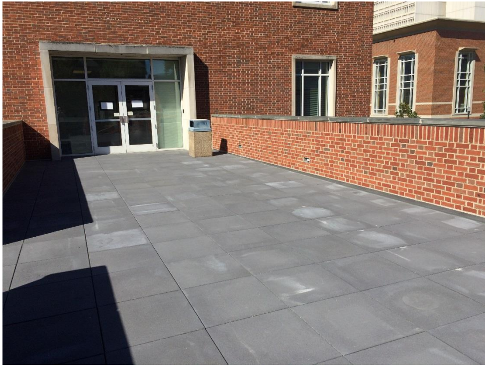
EUC Bridge Repairs
