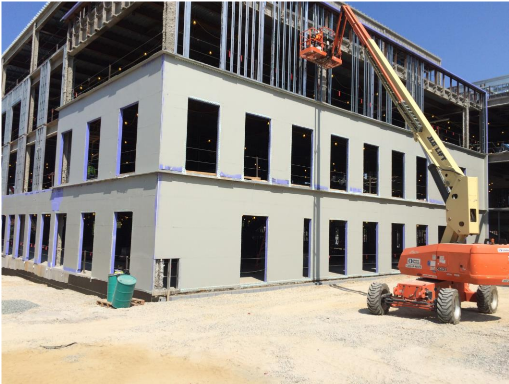
Southwest corner facade in progress. Metal studs and sheathing shown.
