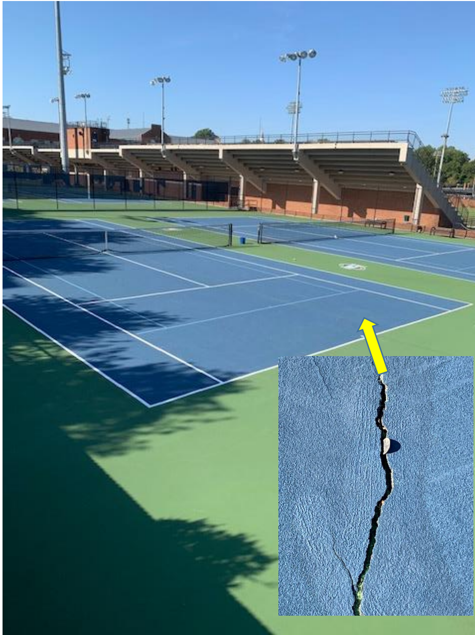
Crack repair of the first six (6) courts in progress.
