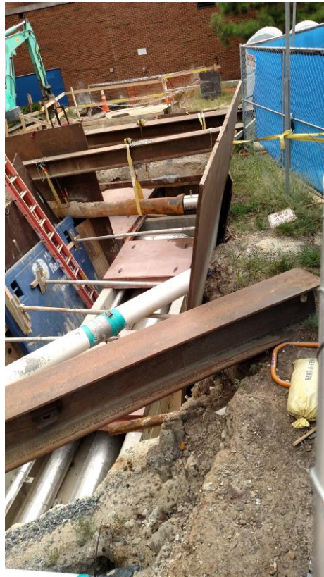
The new steam line being installed between Forest and Stirling Streets.
