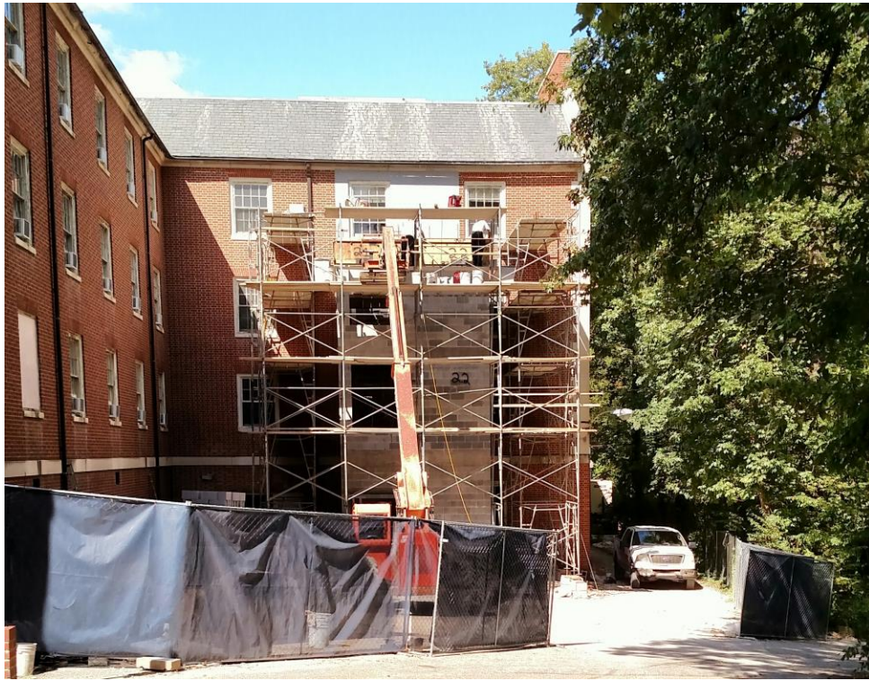
New elevator shaft in progress.
