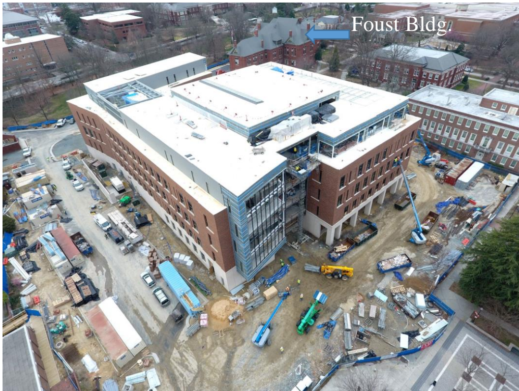
Southwest aerial view of building and site.
