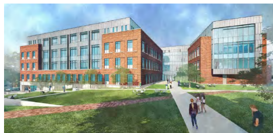
New Nursing and Instructional Building
