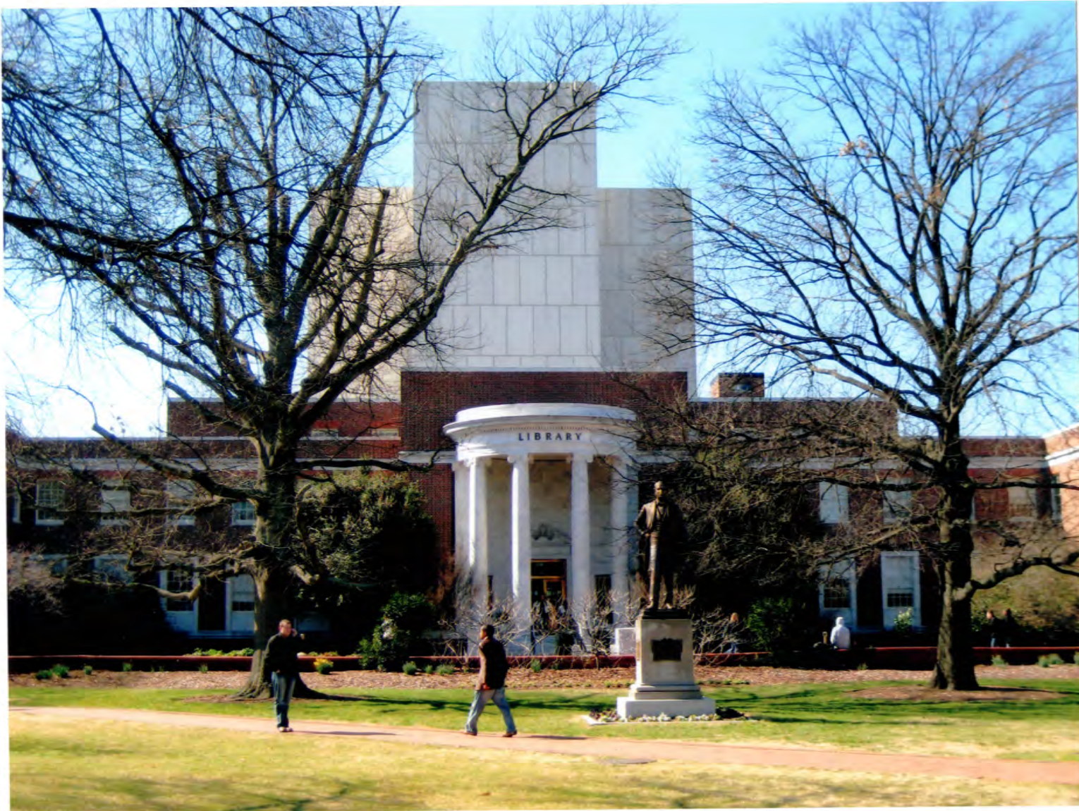
Elevator Upgrades Jackson Library UNC - Greensboro
