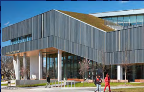
Main Library Addition and Renovation Durham County, North Carolina
