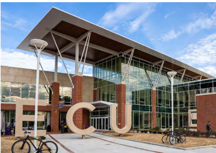
New Main Campus Student Union Commissioning
