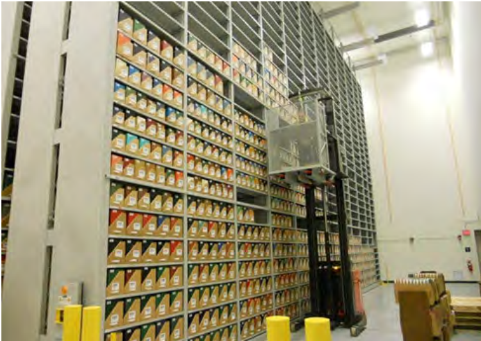
Off-Site Library Storage Facility Renovation Commissioning
