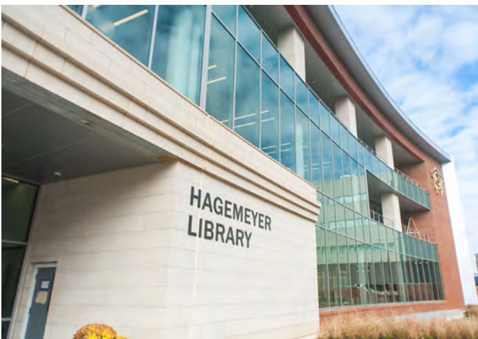
New Parr Center Commissioning, Hagemeyer Library
