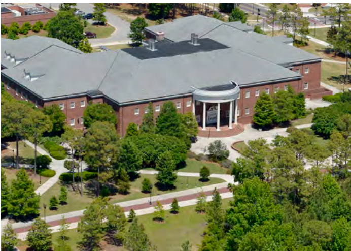
Dobo Hall Laboratory Building Renovation and Re-Commissioning
