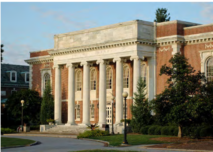
Lilly Library Addition and Renovation Commissioning
