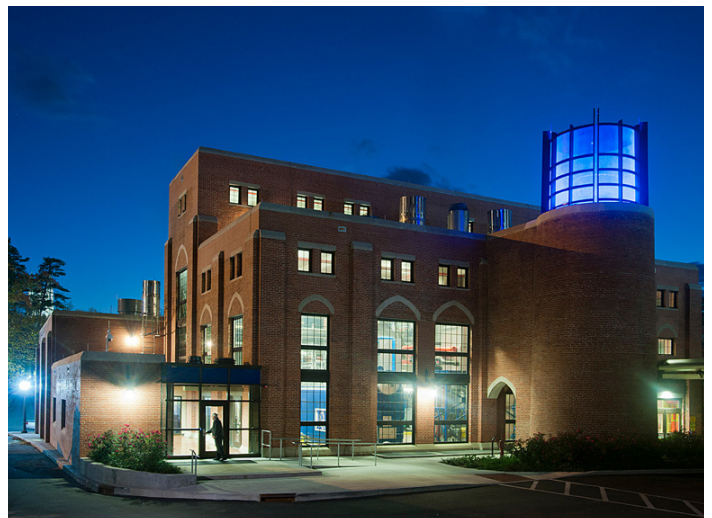
West Campus Steam Plant Renewal and Conversion / Duke University
