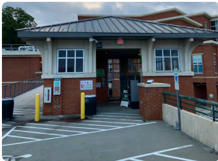
UNCC Union Deck Elevator
