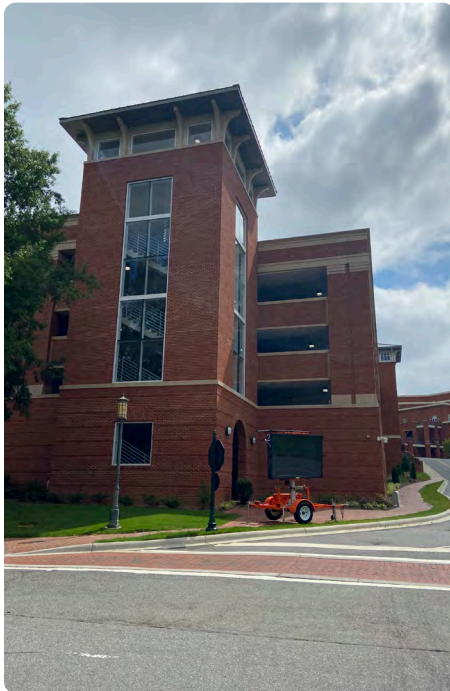
UNCC Union Deck Elevator
