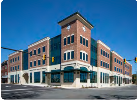
RCC Robinette Classroom Building
