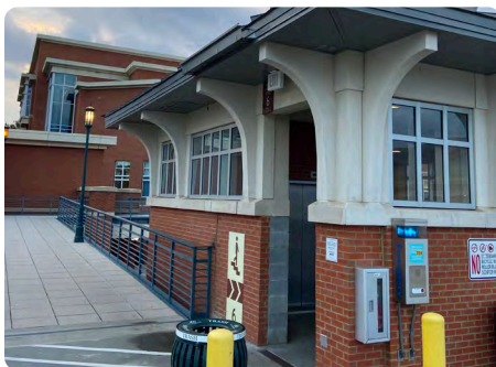
UNCC Union Deck Elevator
