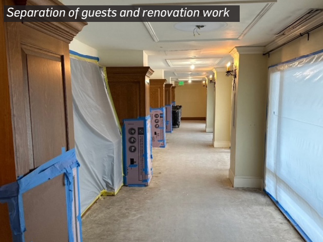
Biltmore Inn Renovations
