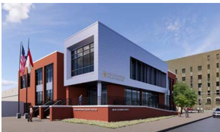
Law Enforcement Building (In-Construction) Guilford County Size: 57,000 SF // Cost: $26,600,000
